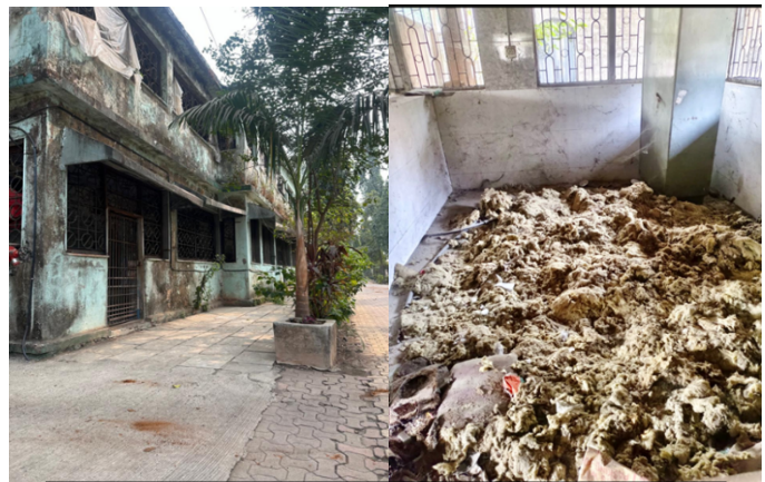
ABANDONED BUILDING AND POORLY USED SPACE INSIDE THE HOSPITAL
