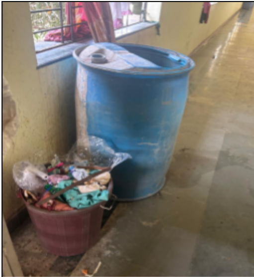
The dustbin has different types of waste (clothing and plastic) disposed in it. It has also been placed near an open water tank. This could lead to the contamination of the water.
