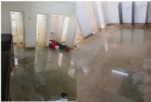
Ekalavya School boys Hostel Washroom and Bathroom
