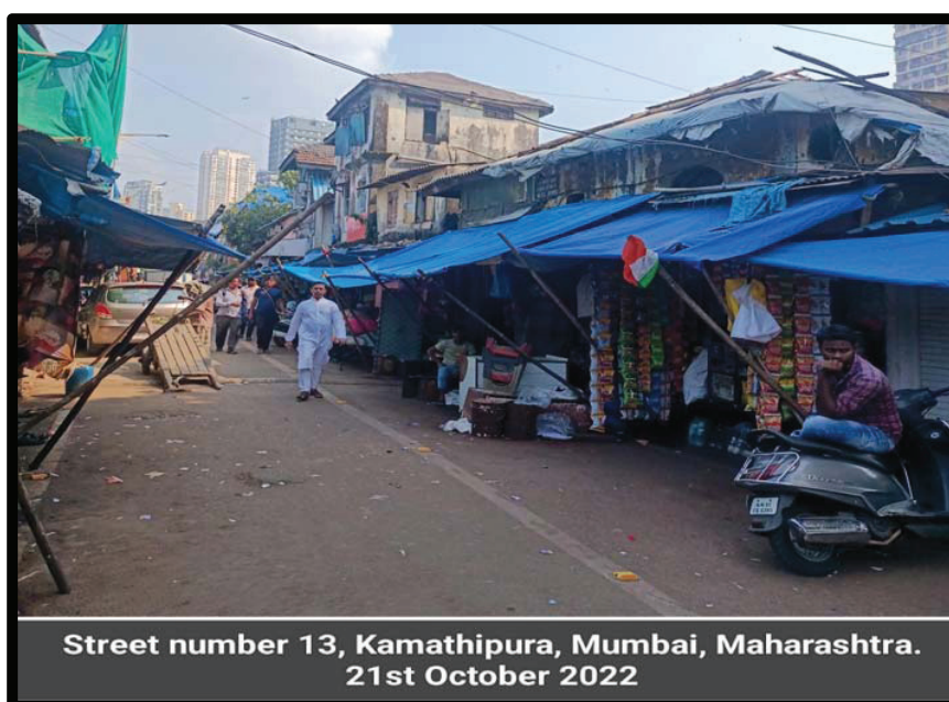
Photo reference: The dilapidated condition of houses in kamathipura.
